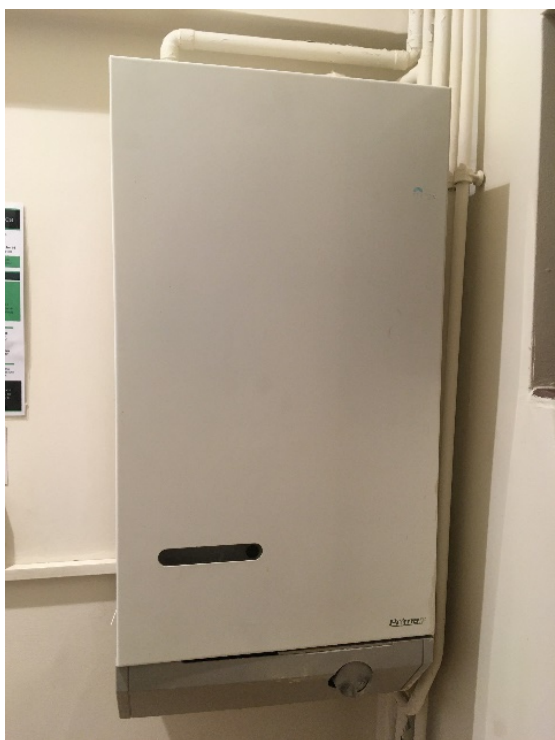
Existing Potterton PrimaF Gas Boiler
