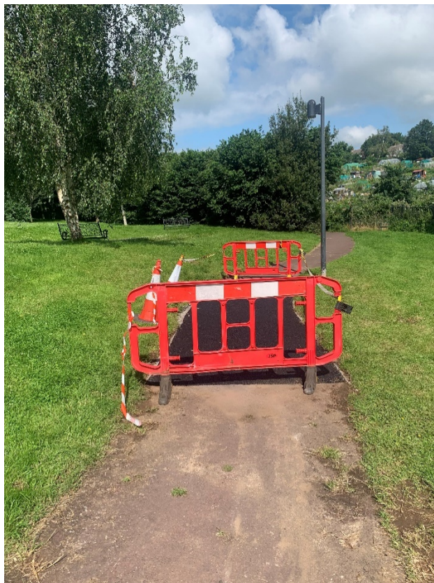
Figure 7: Backfilled with layer of terram and compacted stone and retarmacked
